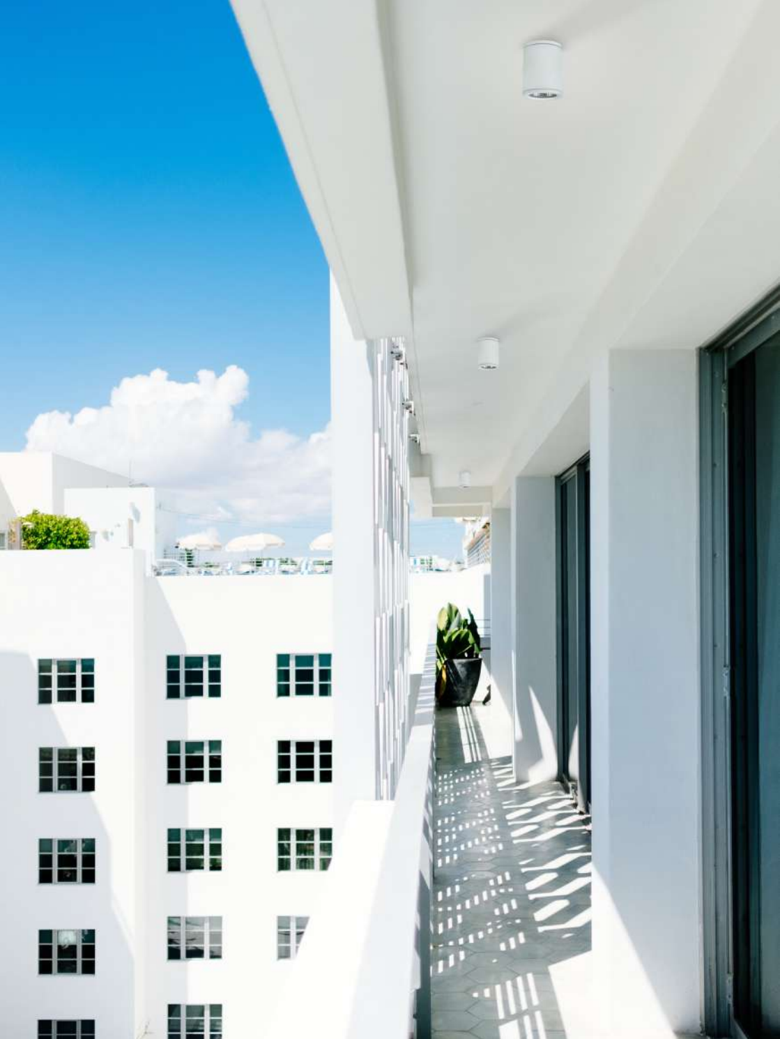
OUTDOOR - CEILING FIXTURES
